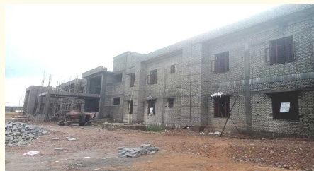
Construction view of Building COA, Hindoli
