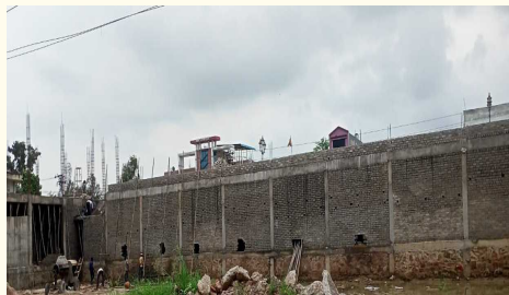
Halls and sale counters construction work
