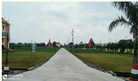
CC Road construction
